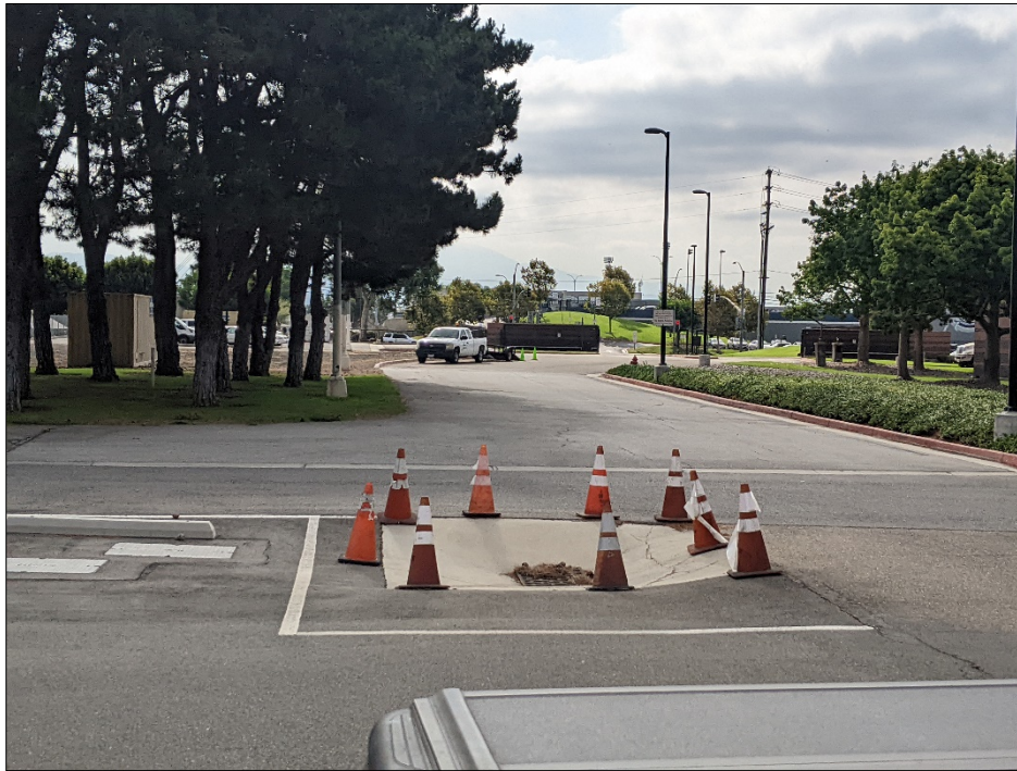
Photograph 4: Proposed and existing eastern access road alignment. View to the east.
